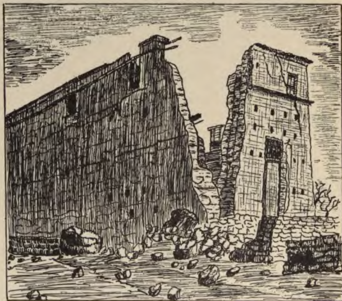
FIG. 6.—The Cathedral of Paterno in the Basilica damaged by the earthquake of 1857 (after Mallet).
